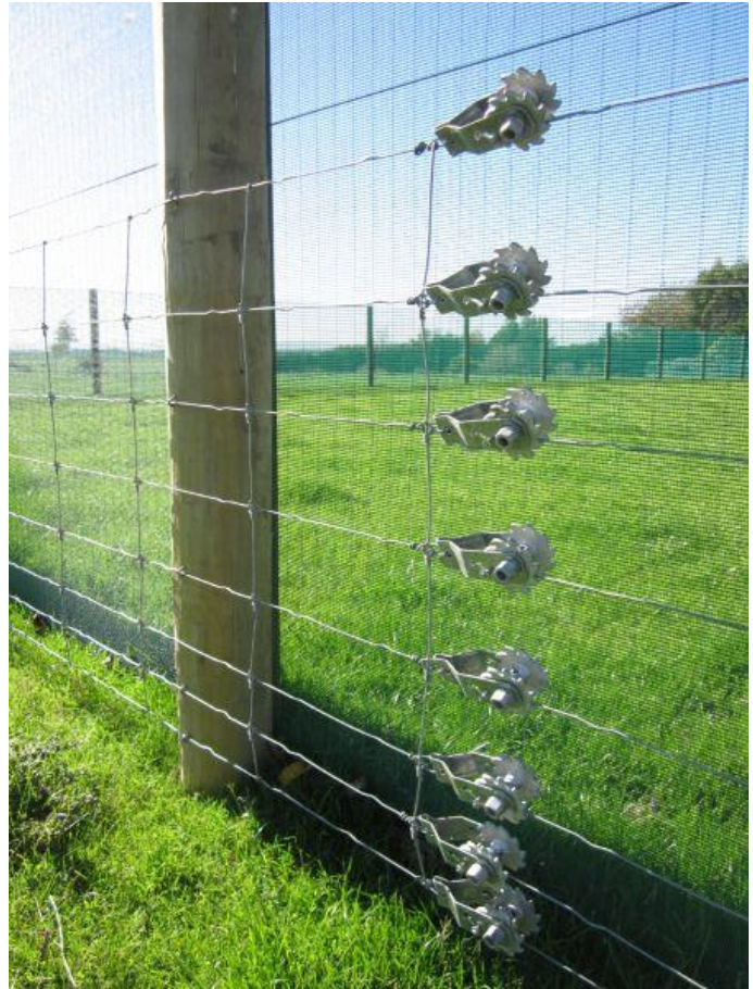
Netting fences use posts with the vertical and horizontal wires designed to withstand sustained stock pressure in holding areas
