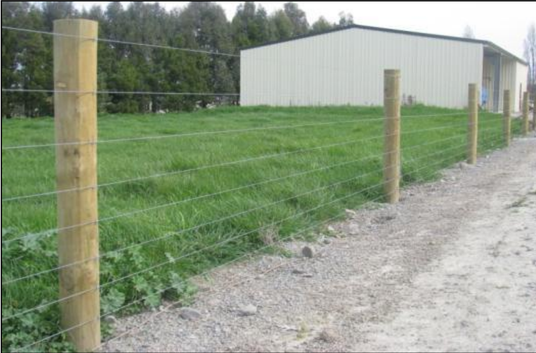
Post and wire fence with round posts spaced at 3 - 5 metres and 8-9 wires of 2.5mm high tensile wire.
