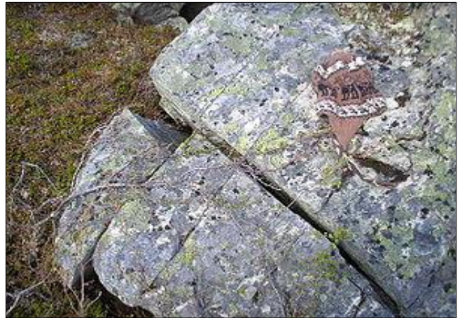
Figure 2: Rock cracked by freezing ice
