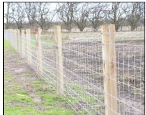
This netting fence features netting, posts, wires and is designed to withstand sustained stock pressure in holding areas.
