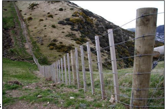
Figure 3 - Multi wire, multi batten (Post and Batten fence) with 1.8mtr No1rnd posts spaced at 4 metres. 5 battens between each post and 7 wires of 2.5mm high tensile wire with spacing as shown
